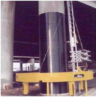
Figure2. Application of FRP for seismic retrofitting of RC columns
