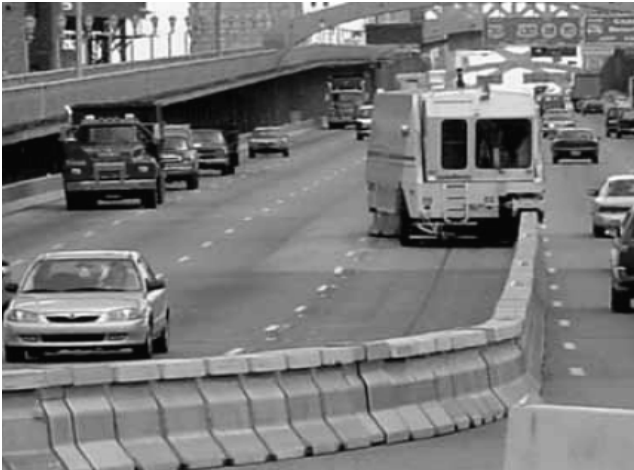
Figure 4. Concrete movable road barrier and BTM (Source. ITS International, 2010)
